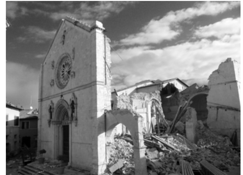
12. Destroyed San Benedetto Church, Norcia (Italy), Norcia earthquakes, October 2016.
